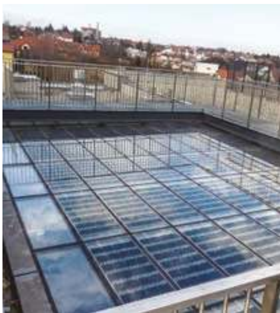
Rzeszów / National Archives / NoFrost modules installed in a skylight
