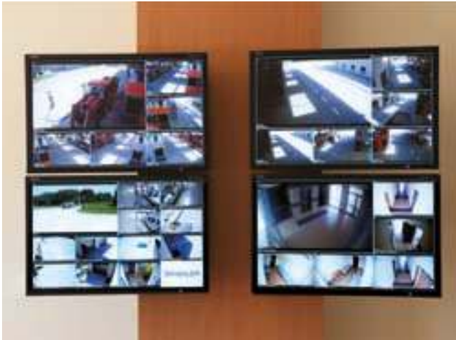
Budomierz / Roadway State Border Checkpoint – video surveillance
