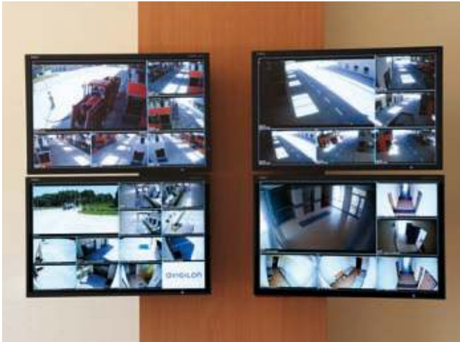
Budomierz / Roadway State Border Checkpoint – video surveillance
