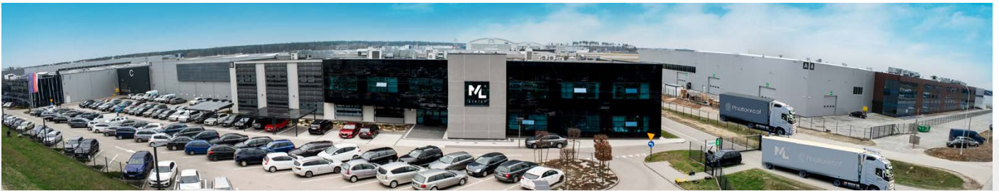
Production plant with an area of 40,000 m 2 , Zaczernie, Poland.
